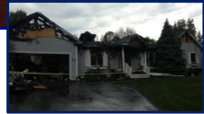
Structure Fire in Stone Ridge subdivision. Reported occupants still inside. Everyone got out safely. Engine 12, Engine 11, and Truck 1 responded.
